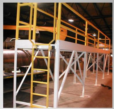
Adding handrails to an elevated platform to eliminate the need for fall protection PPE is an example of engineering controls.
